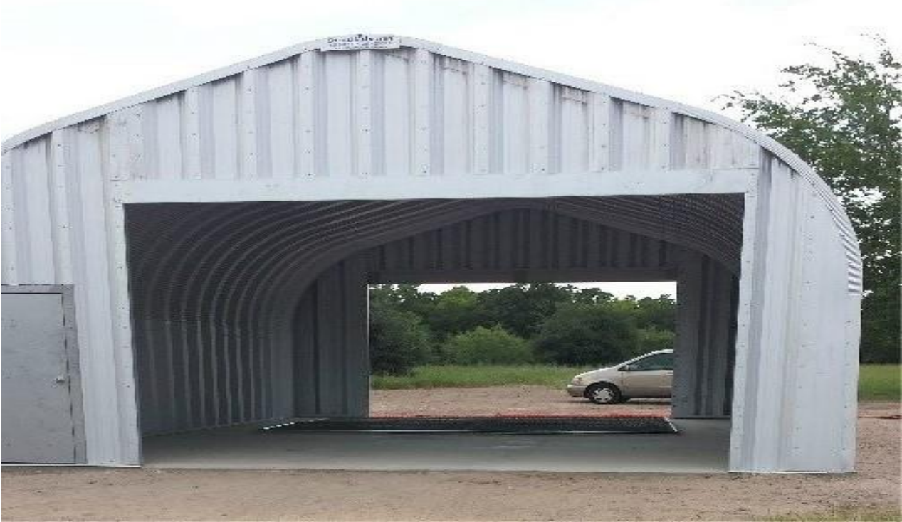
Figure 4: Flywheel Test Facility
